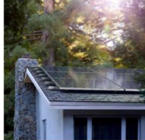
Premium Roof + Solar Panels
